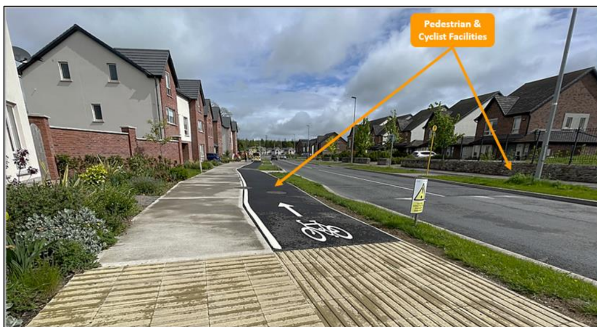
Figure 16.7 View of Hollywoodrath Road (R121) Looking North
