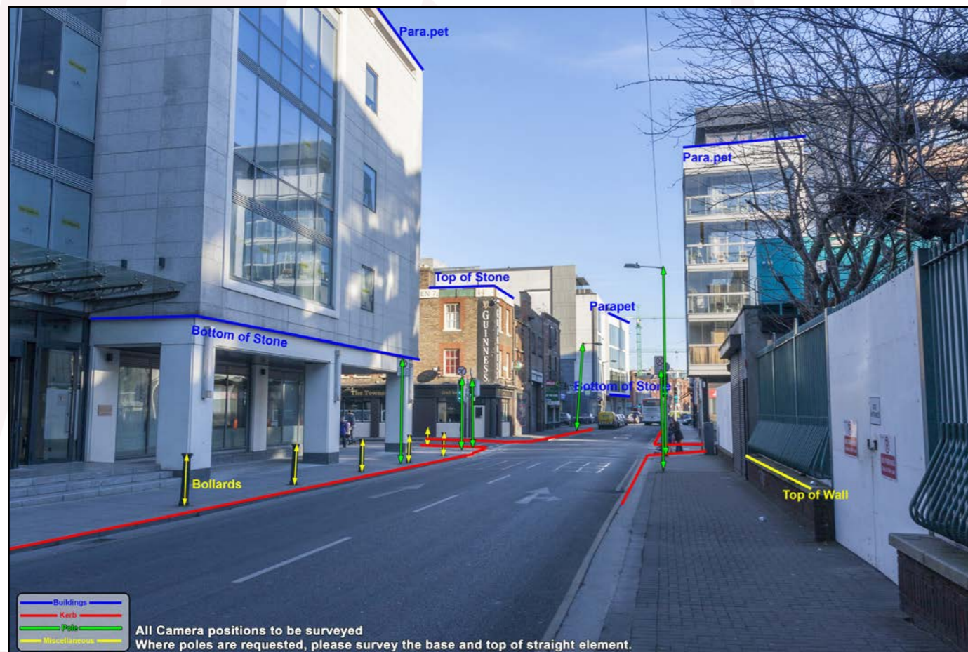
Fig.7: Fixed reference points marked for surveyour.
