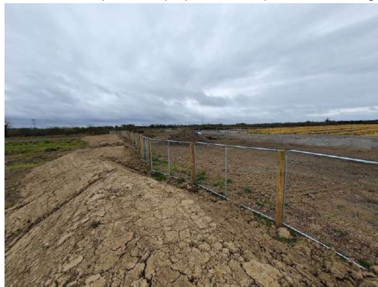
Plate 4 Wayleave for pipeline, facing east
