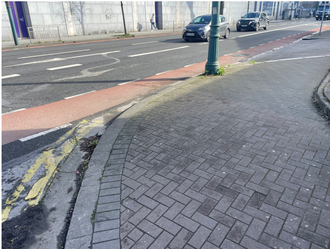
Photo A7: View at NE corner of site, concrete edging to site boundary/kerb edge
