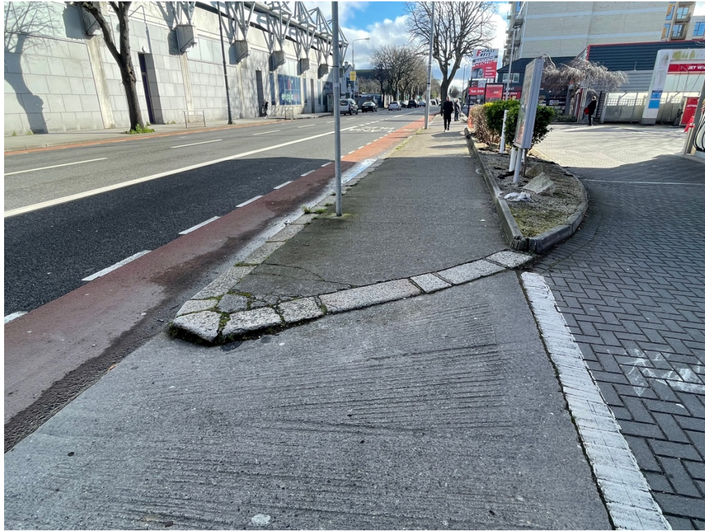
Photo A9: View at northern Donnybrook Road site entrance, granite kerbs to entrance splay
