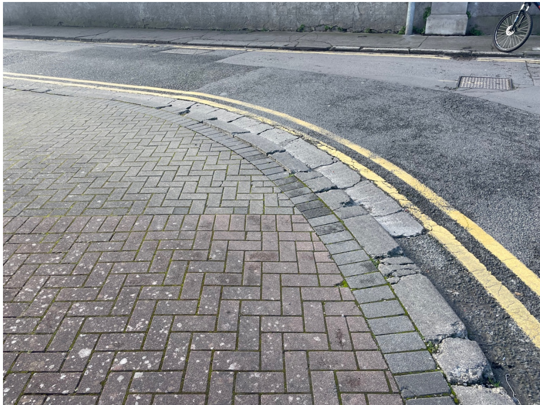
Photo A6: View at northern end of site, concrete edging to site boundary/kerb edge
