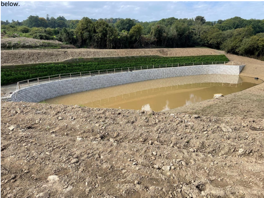
Figure 2.2.1 - Attenuation Pond (under construction)
